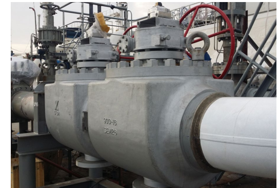
DOUBLE BLOCK & BLEED BALL VALVE for FSRU
